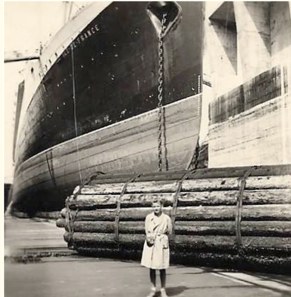
Figure 6: The impressive bow of the ocean liner will be protected by the huge tree trunks bumper when the water level reaches her white waterline.
