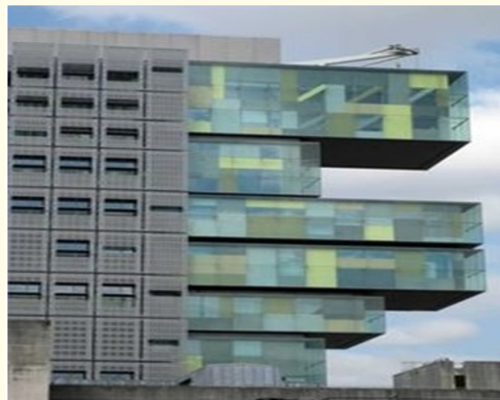
Figure 3: Building with different-frequency consoles for energy dissipation during construction in earthquake-prone areas.
