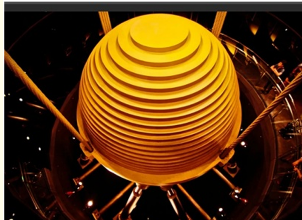
Figure 2: An example of energy damping in the Taipei 101 skyscraper, using an inertial damper.
