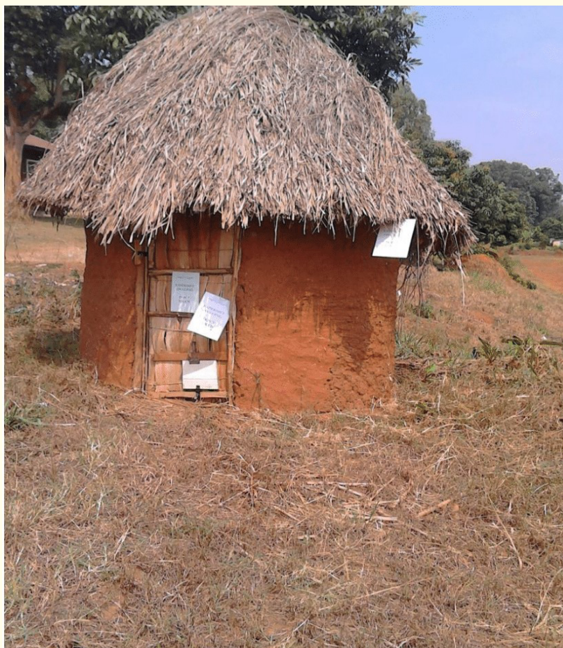
Figure 1: Constructed Storage House (SH).
