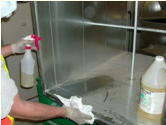
Figure 1: Cleaning and disinfection procedure of air ducts.
